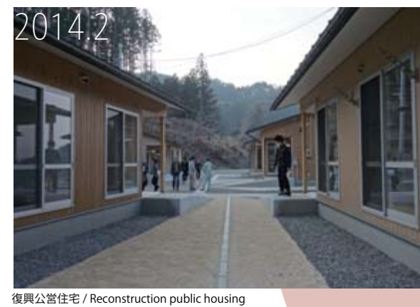
復興公営住宅 / Reconstruction public housing
