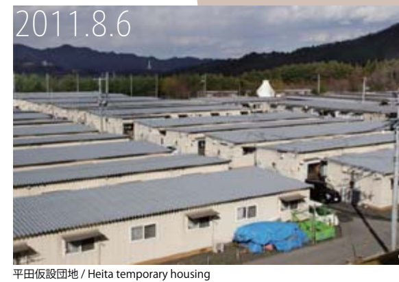
平田仮設団地 / Heita temporary housing
